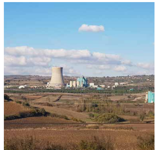
Çan-2 power station in Çanakkale Province (Photo: Sakhalinio – Own work, CC BY-SA 4.0, https://commons.wikimedia.org/w/index.php?curid=111790584 )
